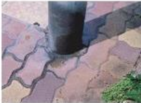
Photo 3. Antifouling effect on surface of photocatalytic permeable block (right).
