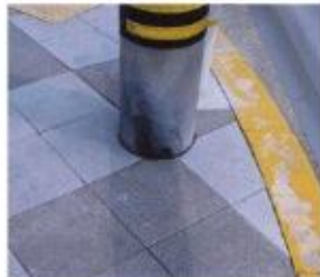
Photo 3. Antifouling effect on surface of photocatalytic permeable block (right).
